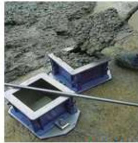
placing of concrete
